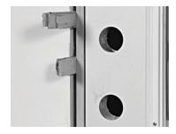
Shim behind the latch-side jamb approximately 8" from the top and bottom of the frame. Install shims until there is an even 1/8"gap between the jamb and the edge of the door slab along the whole length of the door. Shim behind the latch-side jamb just above and below the dead bolt hole, maintaining the 1/8"gap. Pull the weather-stripping away from the jamb and screw 3" installation screws through the jamb and shims and into the stud.
